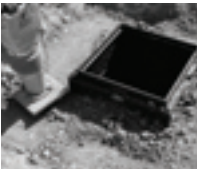
Step 4 Backfill with compacted pea gravel up to 10mm in diameter
