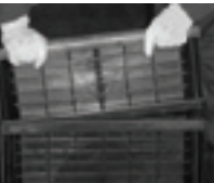
Step 1 Place the access chamber on a solid base to assist assembly of the panels
